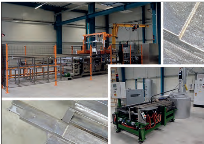
Fig. 14: Automatically tinning plant and casting device at JL Goslar Anoden GmbH
